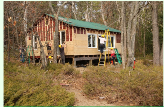
Lasalle Students renovating Woods Greenway cabin
